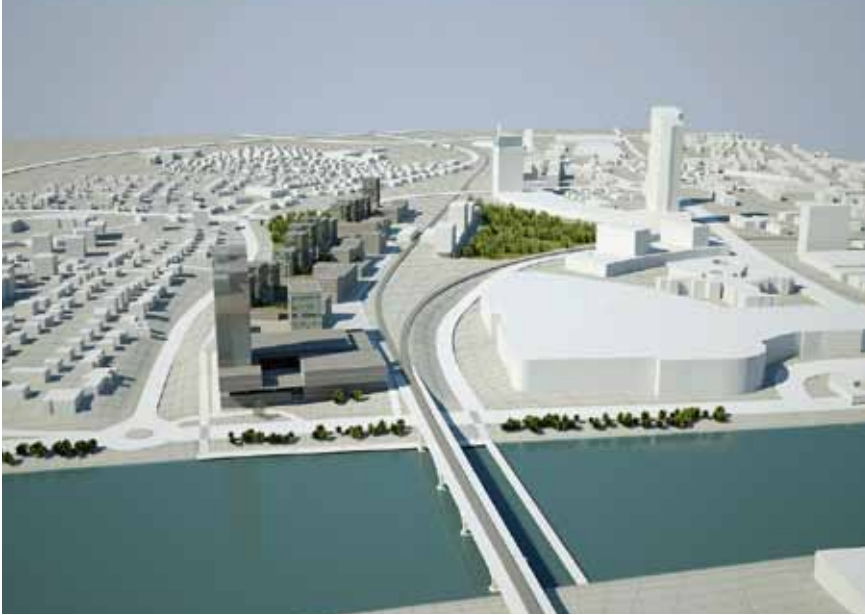
Entwurf des neuen Regionalzentrums am rechten Draufufer Concept for the new regional centre on the right bank of the Drava
