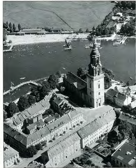
In place of the church of the Holy Spirit – destroyed in World War II – an old people's home was built; the tower recalls the former church steeple.
