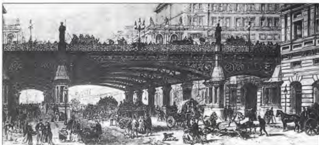
Bild 3: Holborn Viaduct in London, vollendet 1869. (Barker/Jackson, 1983)
