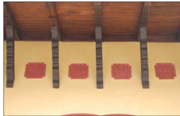
Dachuntersicht. View of roof from below. © Michael Rainer/BDA
