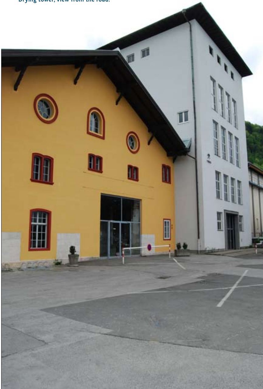
Trockenturm, Straßenseite. Drying tower, view from the road.
